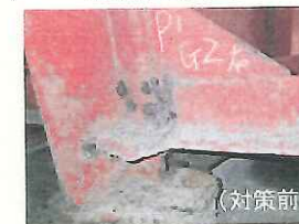
橋梁修繕状況
