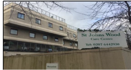
写真1 St Johns Wood Care Center
